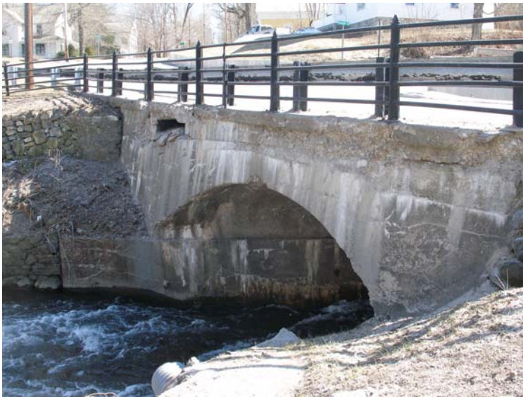
Prior to Rehabilitation
