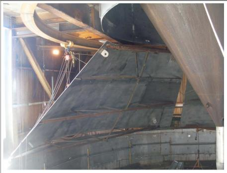
An atmospheric storage tank with a separate tank on top (upper tank operating weight is 600 tons) failed in the transition cone between 21' diameter section and the 40' diameter section. The tank was near failure in the 40' diameter barrel section and lower transition cone.
