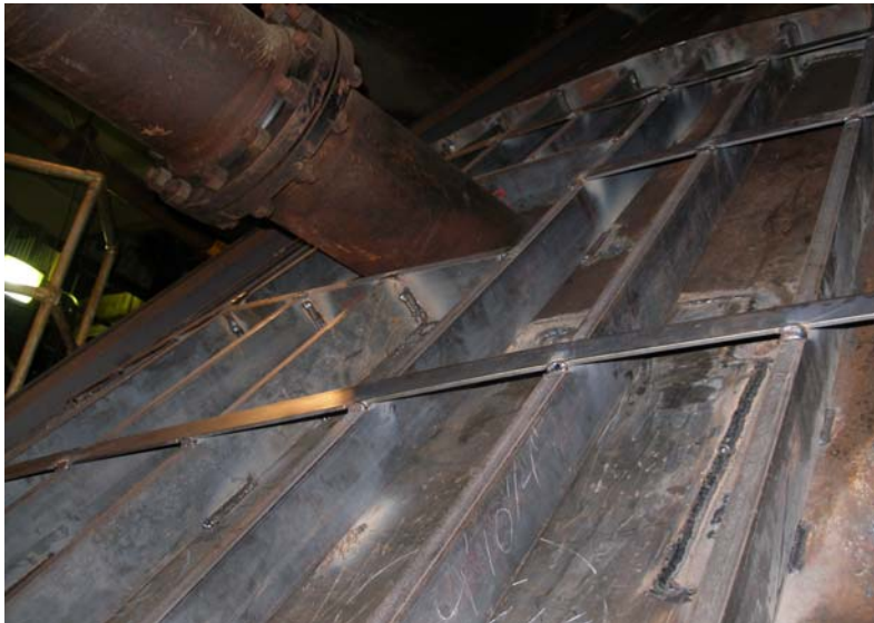
Stiffened Transition Cone with Patch
